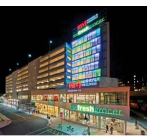
The 1,200-space Wellness Plaza parking garage in New Brunswick, N.J., features a Fresh Grocer grocery store on the first floor and the Robert Wood Johnson Fitness Center on the second floor. The precast concrete structure, designed by TimHaahs, features a corner tower with stairs and four elevators that connect to the adiacent train station's platform. Photo: Steve Wolfe.
